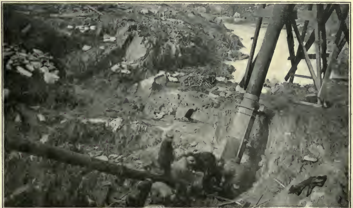
PREPARING TO MOVE THE ELEVATOR.
